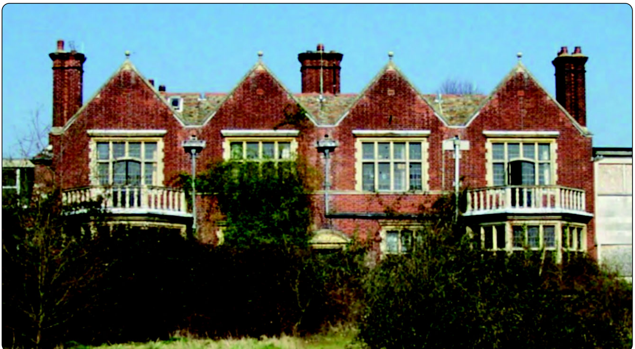
Photo E2. Rear elevation of Houghton Grange
