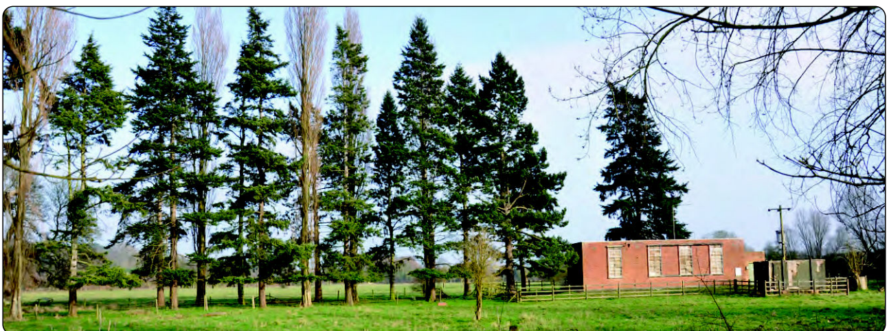
Photo F3. Eastern Pumping Station
